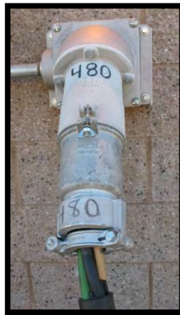
Pigtail plugged into Receptacle
